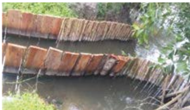
Photo 4 : Installation piscicole (Kouchade M., 2020)
