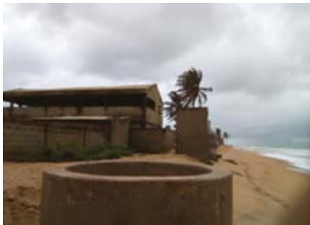
A well now exposed to the waves because the house in which it used to be is destroyed.
