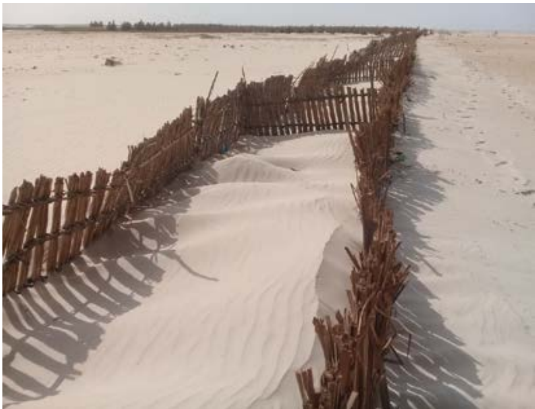
Installation of Typha australis (typhavelles) palisade to fix the coastal dunes of the Langue de Barbarie in the Saint-Louis MPA (WACA FFEM)
